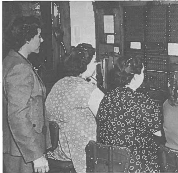
Telephone Company switchboard, Archbold, Ohio. (195?)
