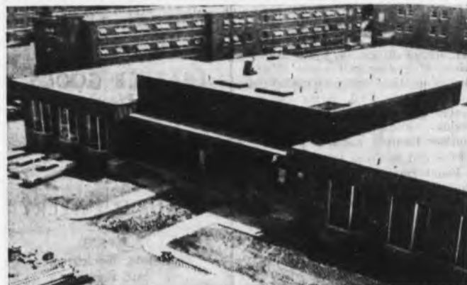
SEPTEMBER 8 IS the completion date scheduled for the new addition to Kohl Hall. Interior painting of the addition is to begin today.
