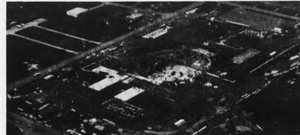
CONSTRUCTION OF THE NEW MEN'S RESIDENCE CENTER is shown in this NEWS aerial photograph by Terry Wolf. Using a Speed Graphic Camera with a 135
