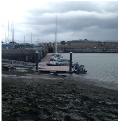
Photo 1. Floating/Pontoon dock area
