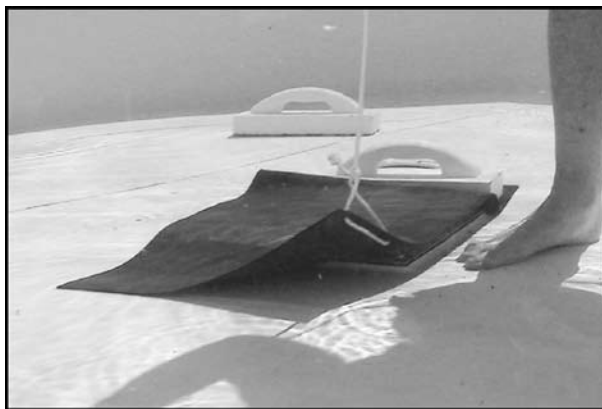
Photograph 8 — Neoprene rubber sheet covering 12" × 12" main drain.
