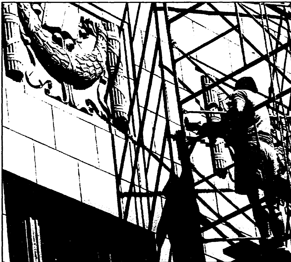
McFall Center is receiving a makeover this summer as employees of George Brothers Building Maintenance of Forest, Ohio, are doing tuckpointing and repairing loose mortar on the exterior walls. They also are cleaning and replacing some of the terra cotta trim.
