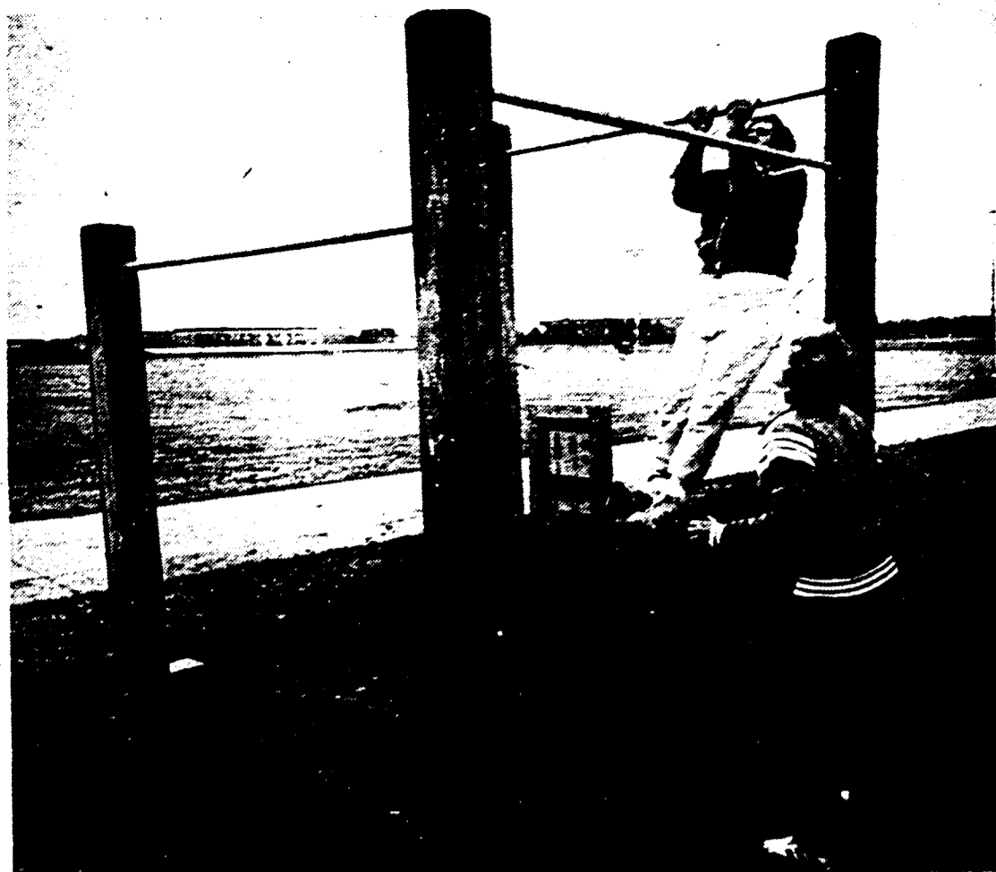
Construction of the University's outdoor "fit trail" is well underway, but weather conditions have prohibited its completion. The trail is being constructed adjacent to the Ice Arena with $10,000 contributed from private sources.
