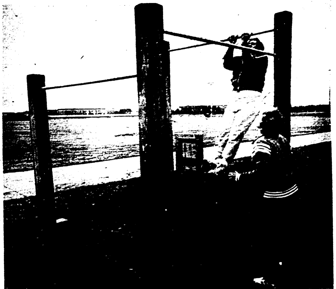
Construction of the University's outdoor "fit trail" is well underway, but weather conditions have prohibited its completion. The trail is being constructed adjacent to the Ice Arena with $10,000 contributed from private sources.
