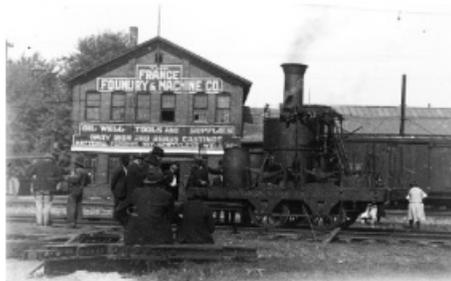
An earlier look back: above right, the "Atlantic," a steam locomotive engine built in 1832 for the Baltimore & Ohio Railroad. The engine is seen in front of the France Foundry & Machine Company of North Baltimore, Ohio, a metal-working shop serving the oil industry and other businesses. The engine may have been coming through the area in around 1926, on its way to an exhibition of old-time locomotives.
