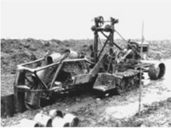
◀ The Buckeye Traction Ditcher Model 301 digs a drainage trench on a farm in 1946. The original company, founded in Bowling Green in 1893, grew to become the largest tile ditching and construction trenching company in the world. A version of the machine is still in production. The Buckeye Traction Ditcher/Garwood Industries Collection (MS 380) is among the many resources available to researchers at the CAC.
