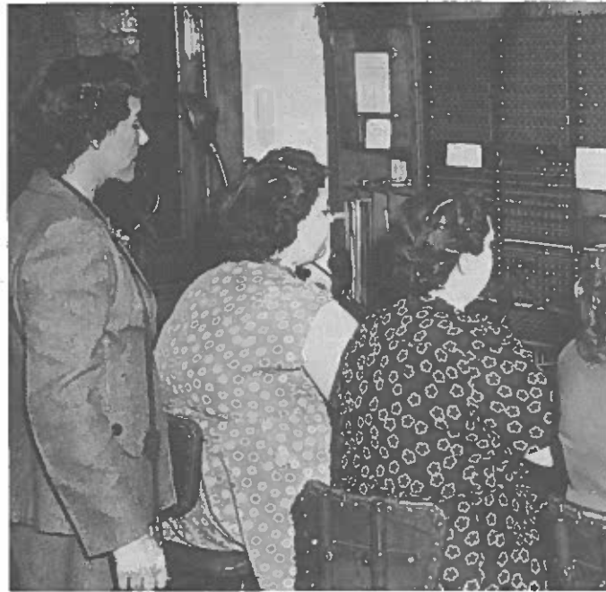
Telephone Company switchboard, Archbold, Ohio. (195?)
