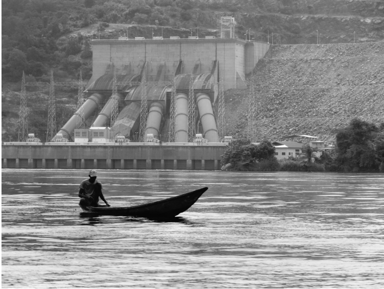
Photograph 2.1: Akasombo Dam. Akasombo Dam is a hydroelectric dam on the Volta River in Ghana. It was initiated in 1961 by Ghana's first president Kwame Nkrumah's administration and completed in 1965. Lake Volta, created by the dam, is the world's largest man-made lake. The World Bank played a major role in funding the dam, along with the governments of the US and the UK.
