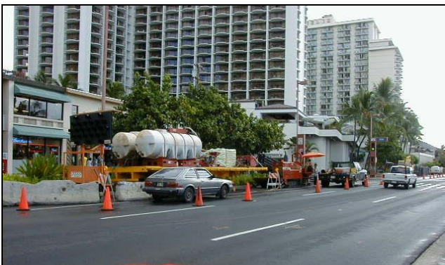
Figure 8 Minimum impact of HDD operations on the businesses, hotels, and traffic
